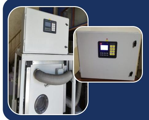
Mitsubishi GOC PLC based Control Panel for EV Motor Testing and Soaking Chamber for Automobile MNC
