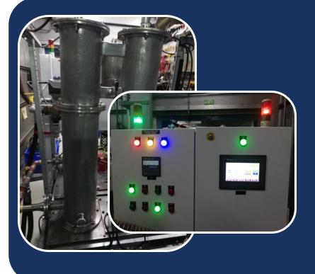
PLC HMI based Control Panel for Engine Coolant Temperature Thermal Shock Unit for Engine Testing in Automobile MNC
